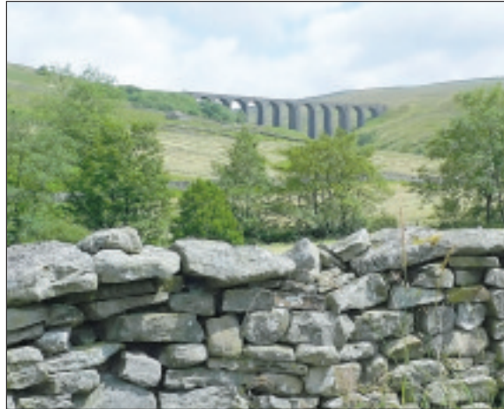
■ One of 17 viaducts on the famous Settle to Carlisle railway, in Dent
